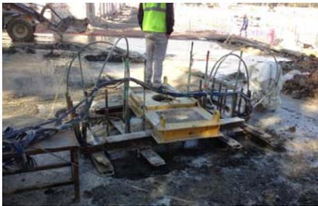
*Completely installed cage instrumented with O-cell assembly, strain gauges and TIP strings*
