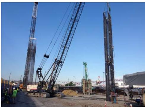
Cage placement with O-Cell assembly
