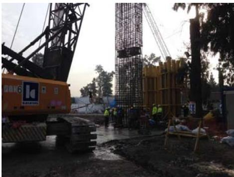
Cage placement with O-Cell assembly
